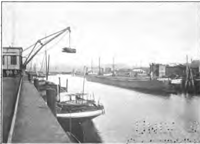
LOADING IRON TIES INTO A BARGE FOR EXPORT AT RUHRORT
